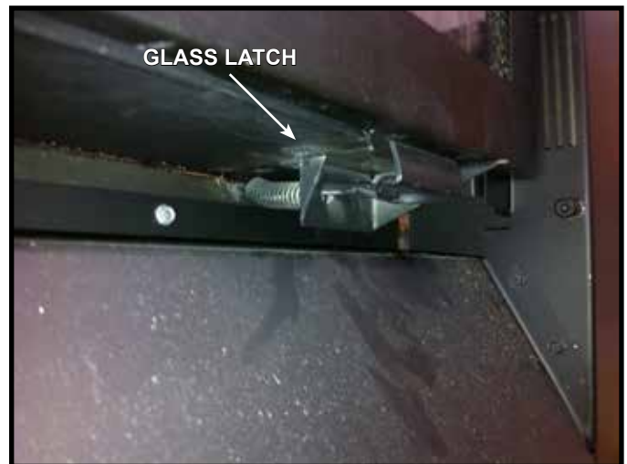
4.4 Glass Latch Detail - Exterior Side
